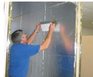
Figure 97. Installing unbaffled return air flow through wall grille.
