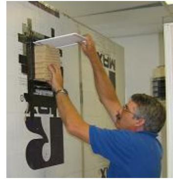
Figure 96. Installing sound baffled return air flow through wall insert made by Tamarack.
