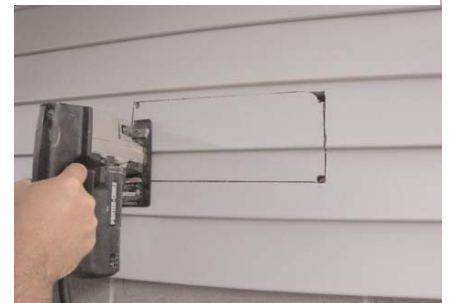
CUT HOLE ALONG MARKED LINES.
