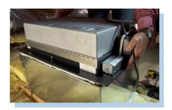
The **Muffler** is an insulated, raised frame plenum box. Engineered to raise select Tamarack brand Whole House Fans 12 inches off the attic floor joists, eliminating the need for joist cutting and reducing fan
