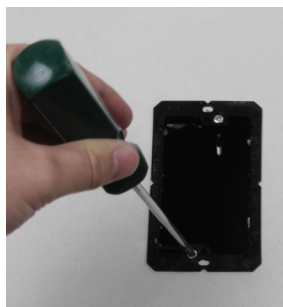
Place the mounting bracket and secure its locking tabs by tightening the silver screws
